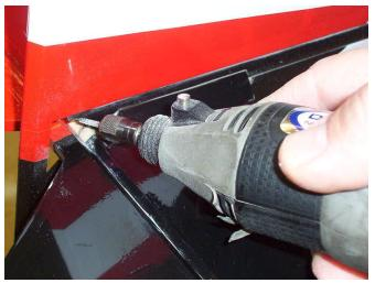
33. Slot the rudder for hinges. I like to use Radio south hinges. I use a 1/4 scale CA hinge for the lower hinge on the rudder.
